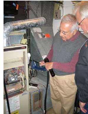
Inspecting HVAC equipment
